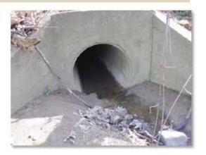
**Problem Summary:** Dry-weather flow with elevated *E. coli* densities was traced to between 7026 and 7041 Greenbriar Drive. Recommend dye testing homes in area to determine improper connections.
