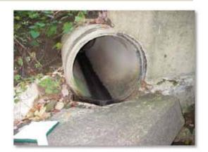
**Problem Summary:** The headwall of the outfall is cracked and has fallen partially northward into the tributary. Additionally, approximately five feet upstream of the outfall opening, the storm sewer pipe has completely separated from the remainder of the pipe and flow is discharged into the ground through the crack and not through the opening of the outfall. The concrete headwall and exposed pipes are in the process of being fixed by the City of Mayfield Heights.
